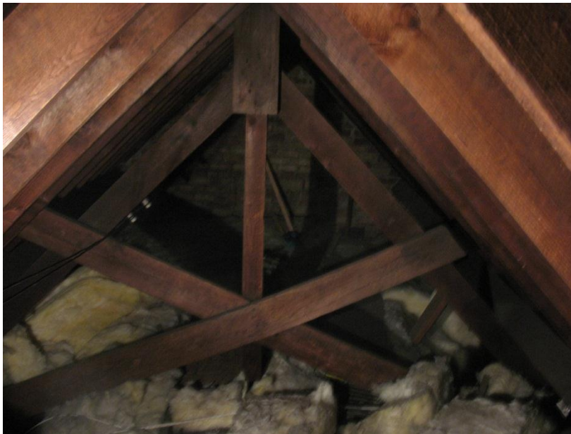
Figure 16. View of altar truss showing face nailed connections throughout.
