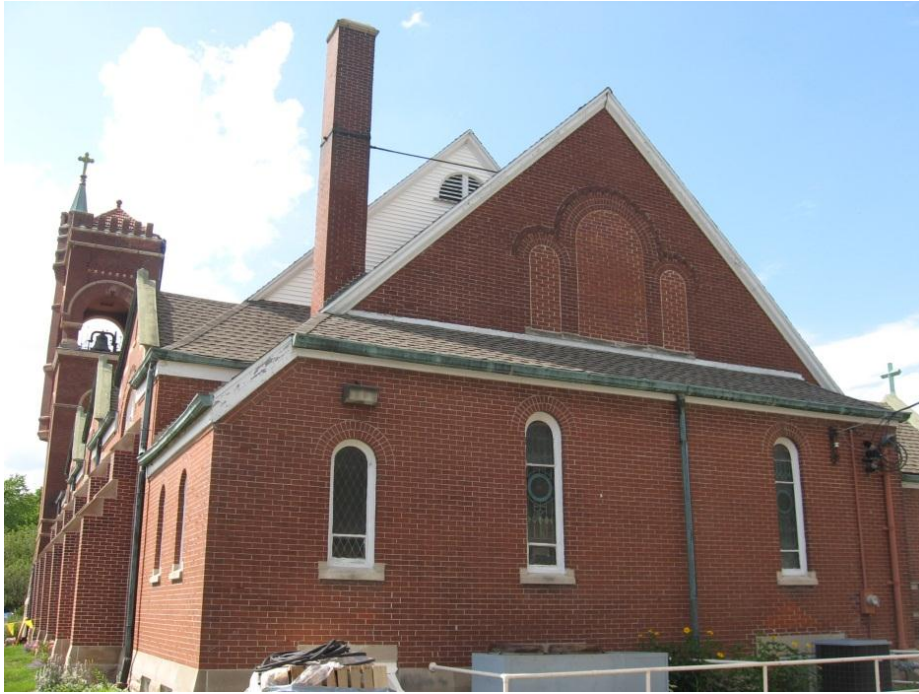
Figure 3. Overall view, east elevation.
