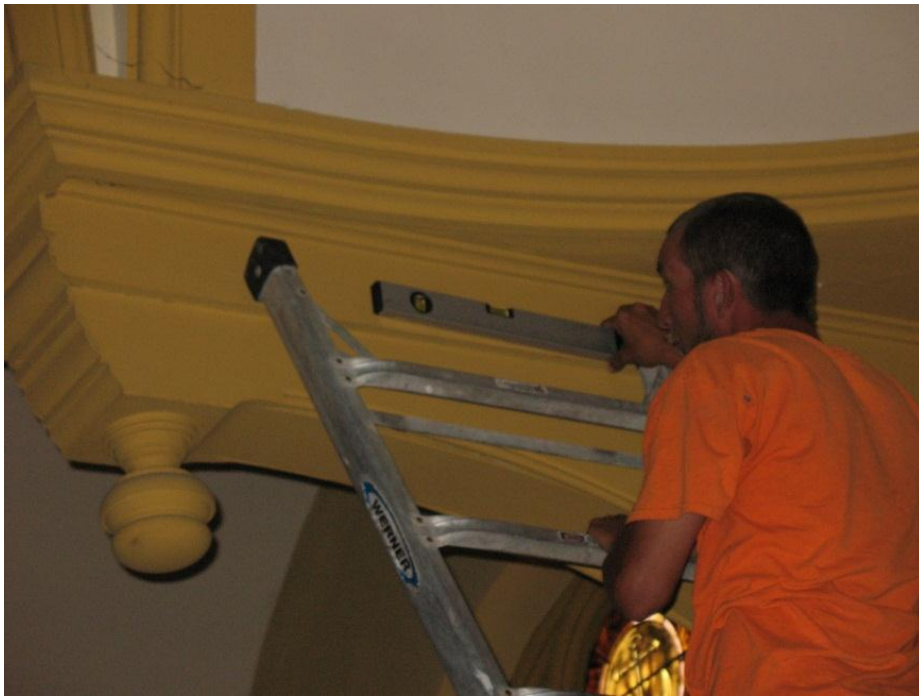
Figure 34. Measuring slope of hammer trusses inside sanctuary.
