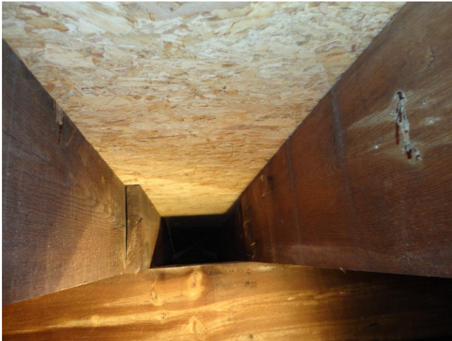
Figure 27. Oriented strand board flooring, north side of sanctuary.
