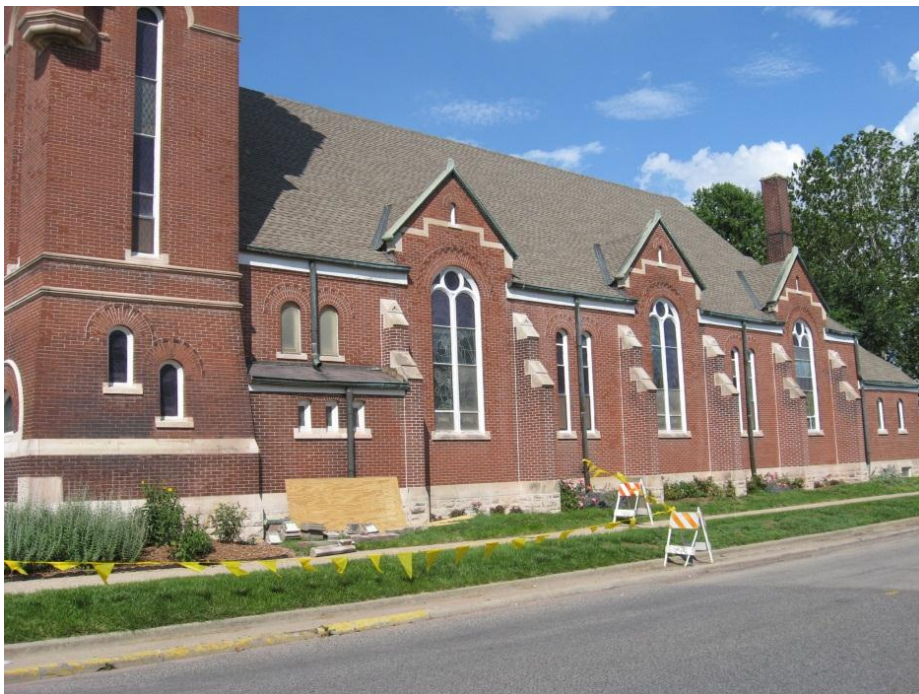
Figure 2. Overall view, south elevation.
