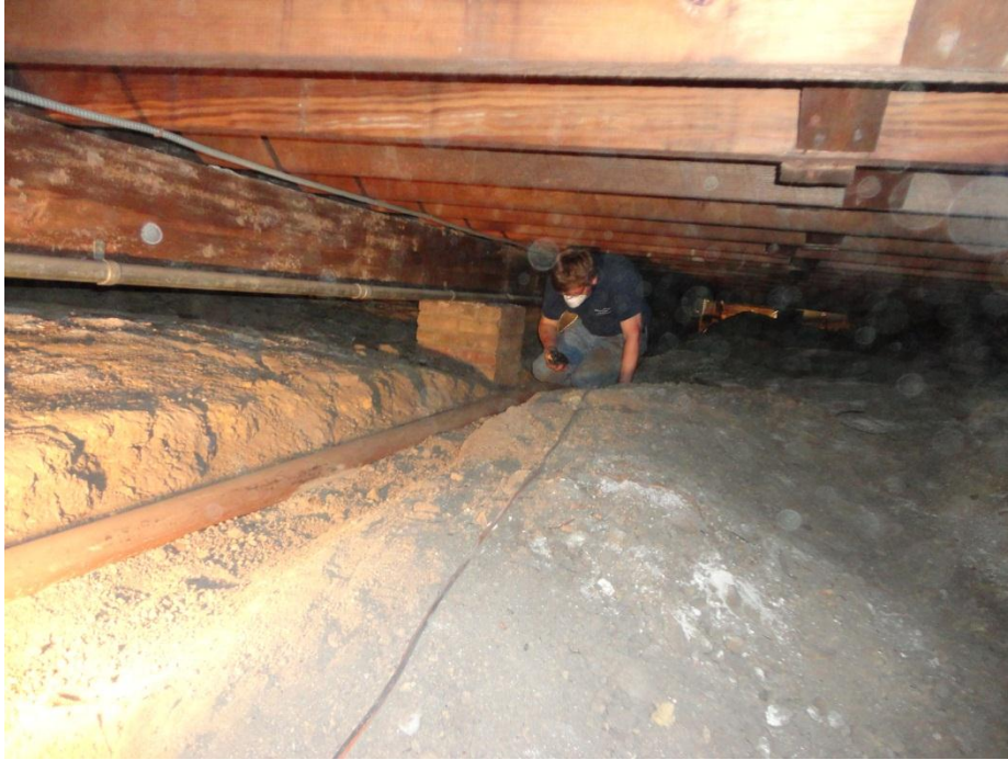
Figure 24. Overall view of joist and beam framing beneath sanctuary.
