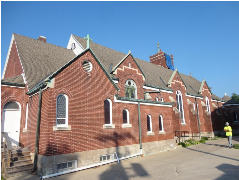
Figure 4. Overall view, north elevation.
